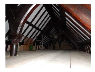
While inspecting the timbers I found several more areas of woodworm holes which Richard inspected. We came to the conclusion that these were all in either dead knots or small areas of sapwood and probably from eggs in the timber at the time of felling. All looked old and inactive. As a precaution I have brush treated these specific limited areas with several coats of penetrating preservative. We intend to take this no further.
